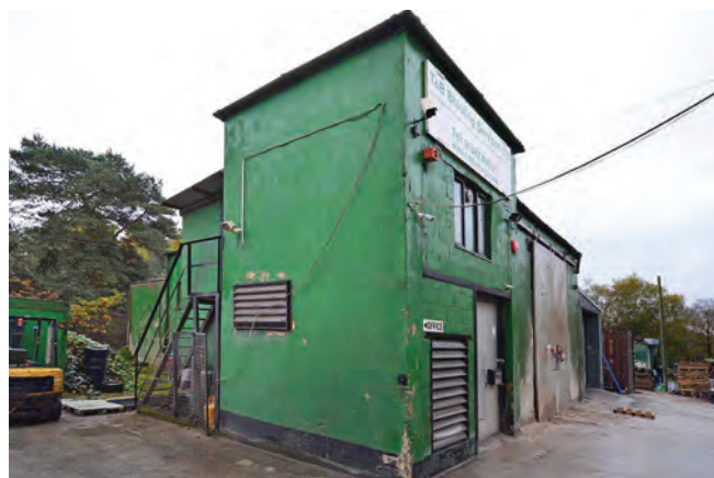
Southernmost of the Generator/Power Buildings
